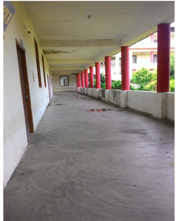
[O]. Corridor of the Lecture Theater Complex
