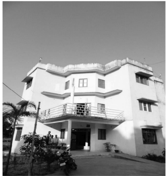
[B]. Front view of Administrative Building
